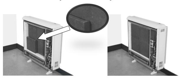
II. - Replace the inner front panel. If the bricks have been fitted correctly you will have no difficulty in replacing the panel. Make sure the bottom edge of the inner panel is inside the front lip of the heater. Please see below:
