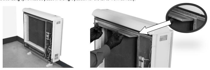
10. - Place the second row of storage bricks with the flat side facing out.
