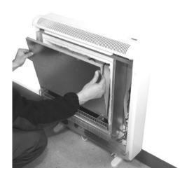
CAUTION In the interior part of this inner panel there is a very delicate thermal insulation MICROTHERM panel. It has to be handled with extreme care. AVOID TOUCHING IT.
